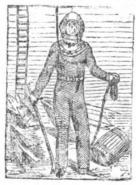
BEG to call the attention of Ship-owners, Merchants, Captains, &c., to the important improvements made by them in the Submarine Helmet Dress and Apparatus, which enables a Diver to remain any Length of Time under Water, for the recovery of Property from Wrecks, Making and Repairing Foundations of Harbours and Bridges, and also for Pearl and Sponge Diving. First Class Medal in the English Exhibition, 1851. First Class Medal in the French Exhibition, 1855.
