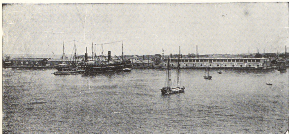
600 ft. STEEL PIER AT WADA. DEPTH AT LOW TIDE 26 ft.
